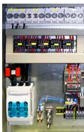
▲ Current transformer in control cabinet
