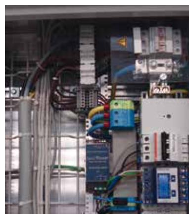
▲ Built-in current transformer in cable duct
